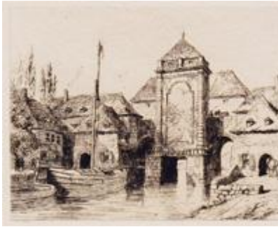
TOURNAI Bridge and Water-Gate
